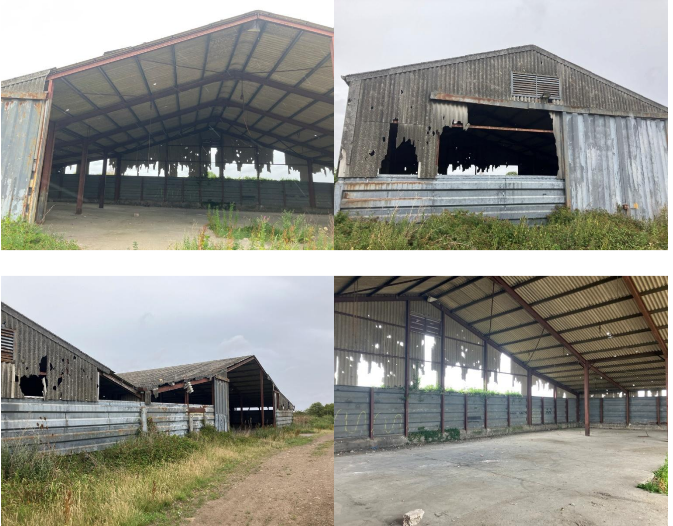
Photograph 1-4: Structure B1 (Internal and External)
