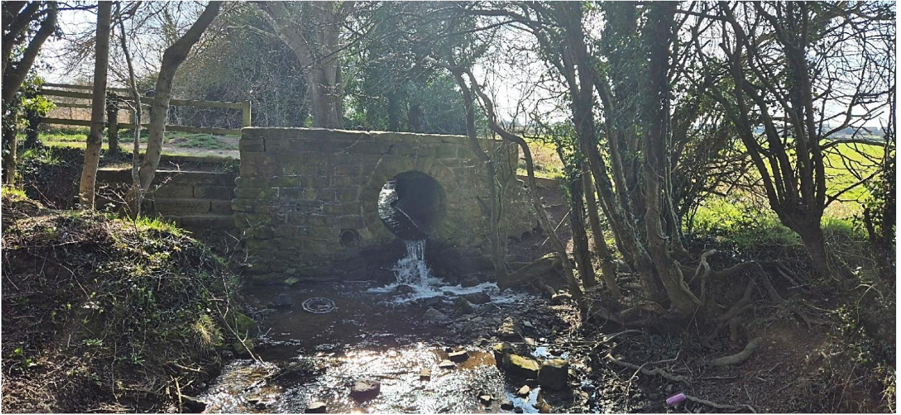
Photograph 9: Structure B3 (External)
