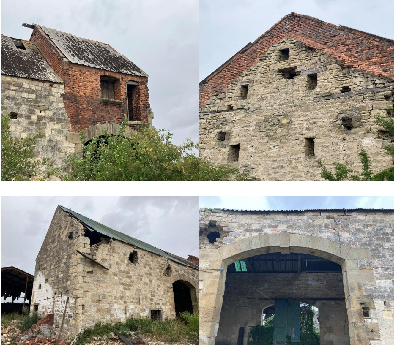
Photograph 5-8: Structure B2 (Internal and External)
